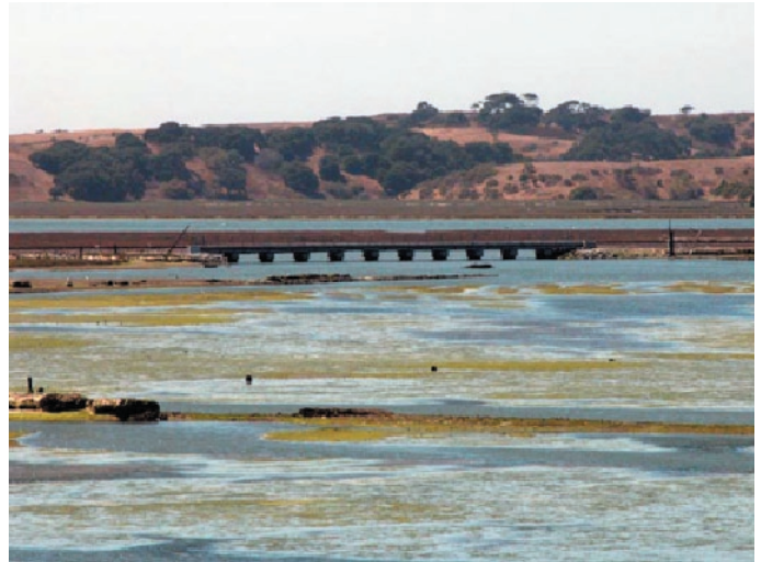
Figure 14. Photograph of the Parsons Slough Marsh complex.
