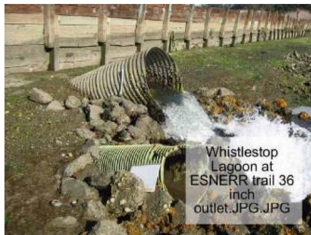
C. The 36-Inch Culvert (Top) and Non-Functional 24-Inch Culvert (Bottom)
