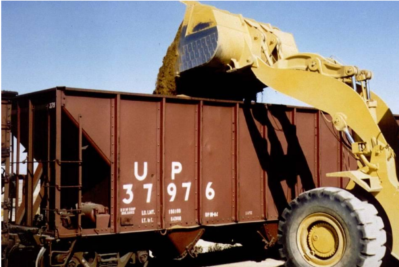
Figure 7 – Sediment Loaded onto a Rail Car for Train Transport
