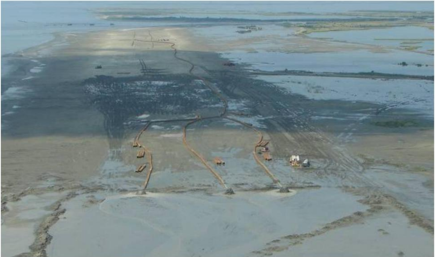
Figure 15 – Hydraulic Discharge Line Layout for Creating Landfill
