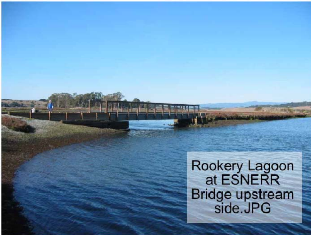
A. Reserve Pedestrian Bridge Looking Northwest
