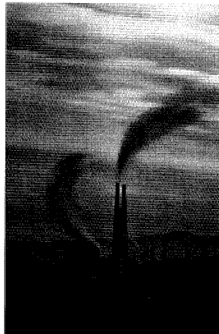
Moss Landing power plant, 1987, with its two 500-foot-tall stacks and multiple smaller stacks. Note stratified wind shear, with onshore flow below 200 feet and offshore flow at higher elevations. Photo credit: Michael Kenna.
